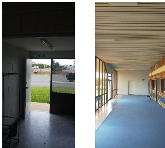
Figure 17 - Exit Signs and No Emergencies
