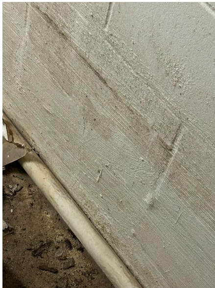
Image 8 – Water-proofing to Inside Face of Basement Wall
