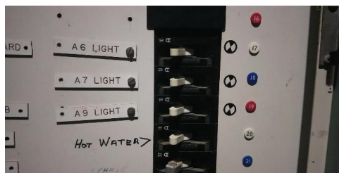
Figure 11 - Circuits without RCDs
