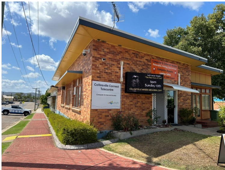
Image 5 – External Elevation of Telecentre
