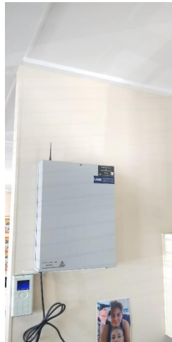
Figure 21 - Integritti Innerange Panel
