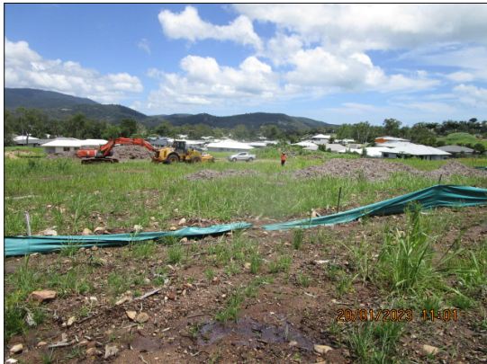
Photo 6 - Inspecting Erosion & Sediment Control
