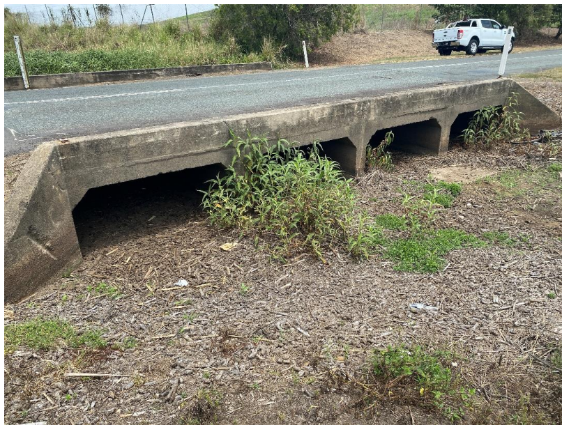
Figure 7 – Existing culverts under Kelsey Creek Rd (subject site's outlet)
