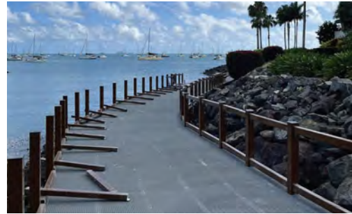
Pictured: Work progressing on Stage 2 of the Airlie Beach Boardwalk Upgrade.
