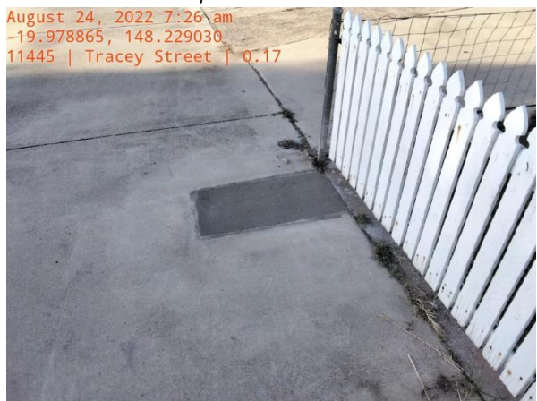
Tracey Street – Footpath Repair
