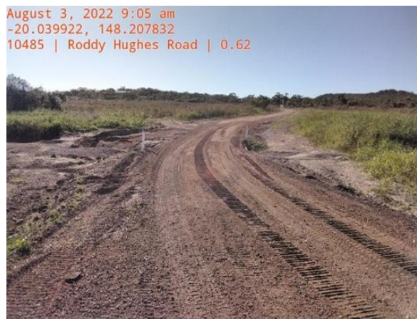
Roddy Hughes Road – Scour Repair
