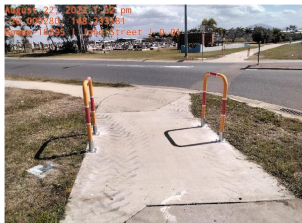
Richmond Road – Replace Guardrails
