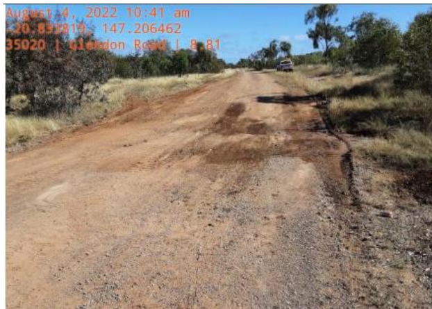
Glendon Road – Scour Repair
