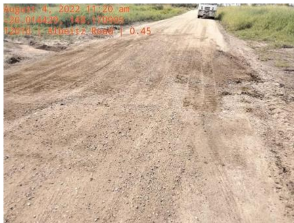
Albeitz Road – Scour Repair
