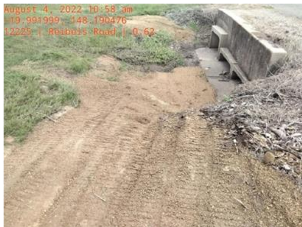
Reibels Road – Scour repair and clearing of Culvert
