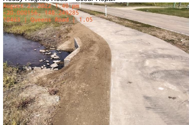
Grading Queens Road – Scour Repair
