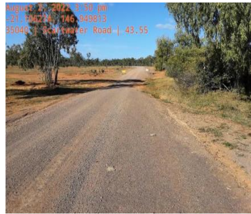
Scartwater Road – Scour repair
