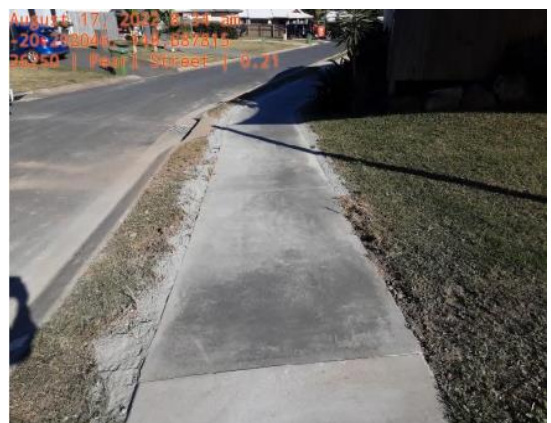
Pearl Street – Footpath repair
