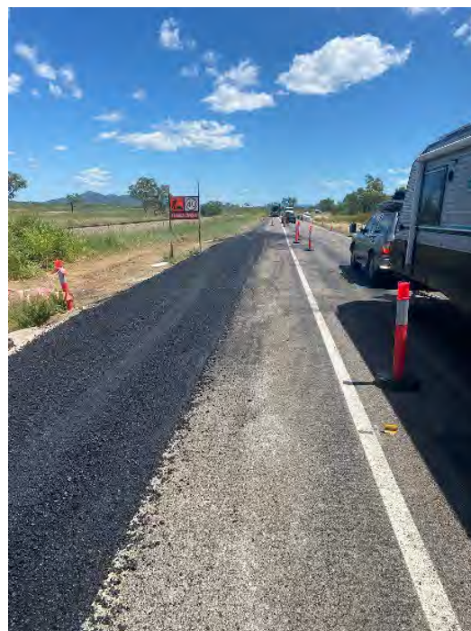
Pavement Repair – 10J RMPC – WBHO Work Sites
