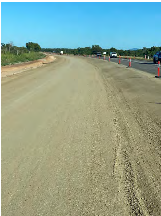
Wedge/Batter Works – 10J RMPC – WBHO
