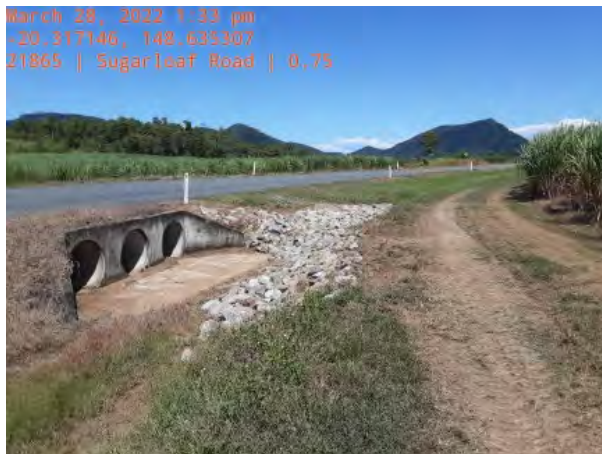
Sugarloaf Drainage works
