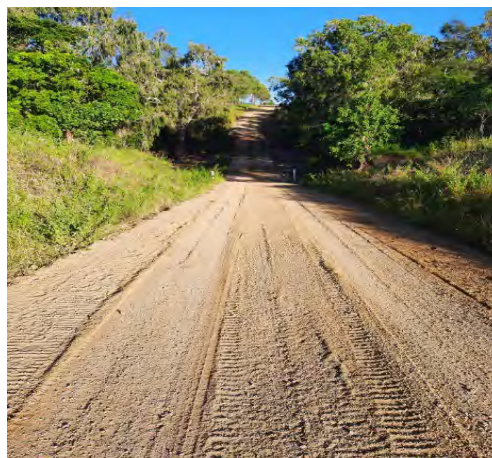
Thurso Road – Scour Repair
