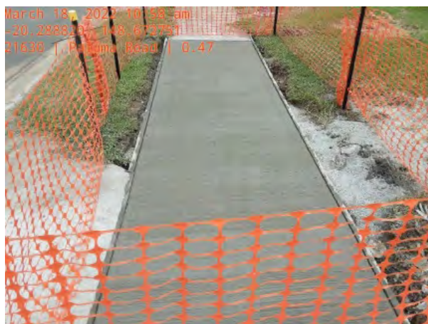
Footpath Replacement works - Maintenance
