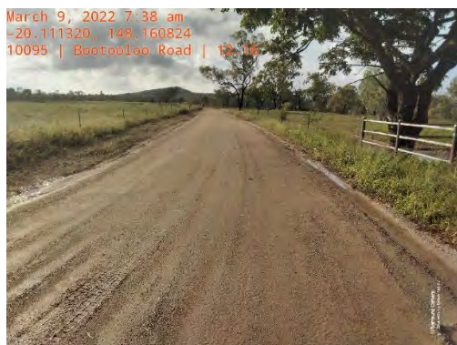
Bootooloo Road – Grading
