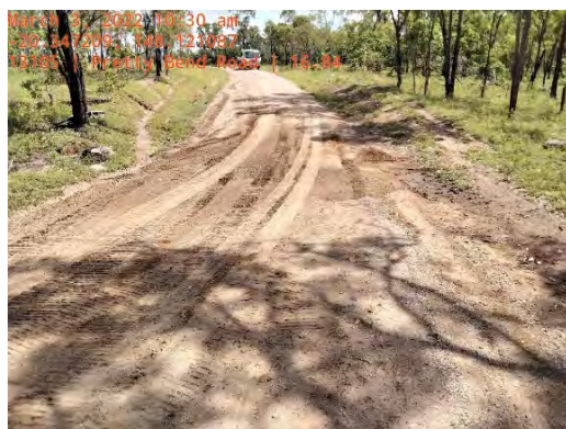
Pretty Bend Road – Scour Repair
