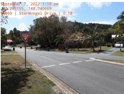
Stormvogel Drive – Refurbish Line Marking
