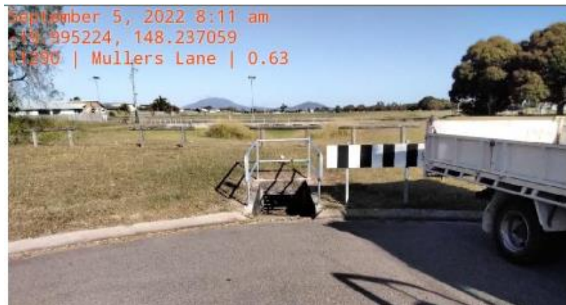
Mullers Lane – Guardrail
