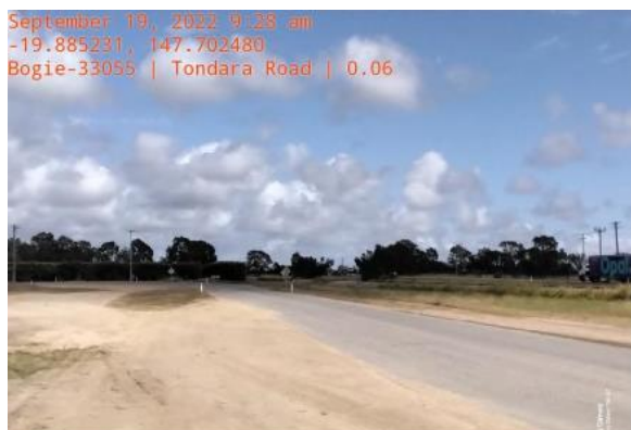
Tondara Road - Shoulder Grading
