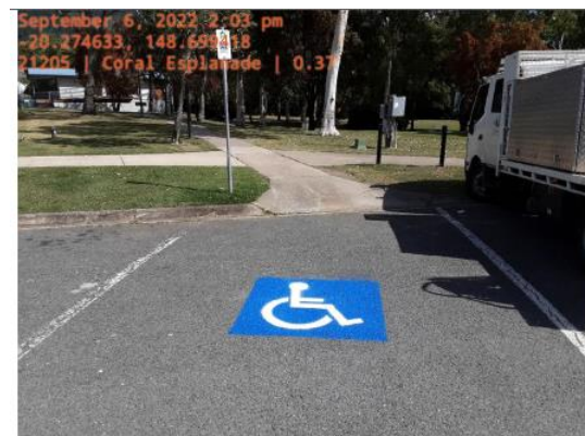
Coral Esplanade – Refurbish Line marking
