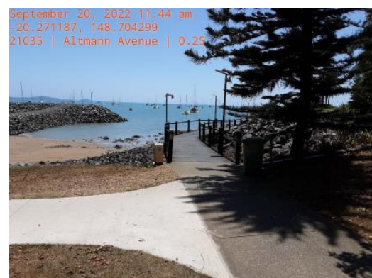
Bicentennial Walkway – Boardwalk Repairs
