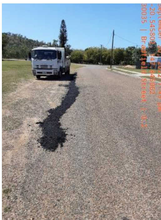
Bradfield Street - Crack Seal Patching
