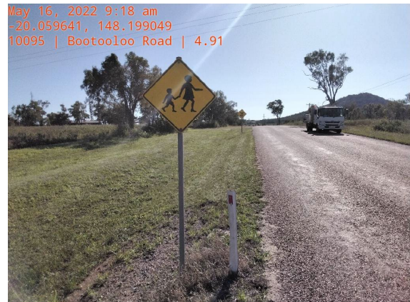
Bootooloo Road – Sign Repair
