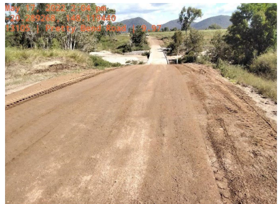
Emergent Works – Pretty Bend Road – Scour Repairs
