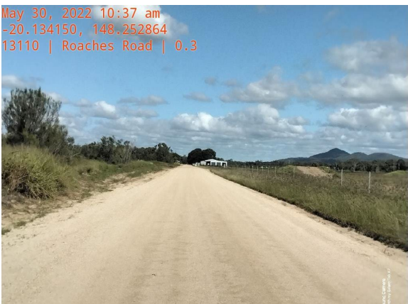
Roaches Road – HFG
