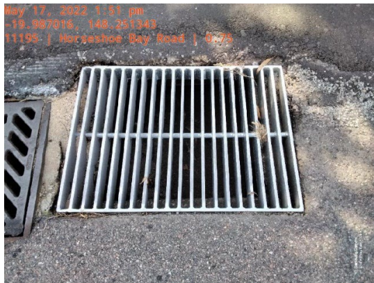
New Grate – Horseshoe Bay Road
