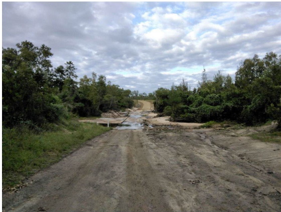
Pretty Bend Road – Vegetation Clearing
