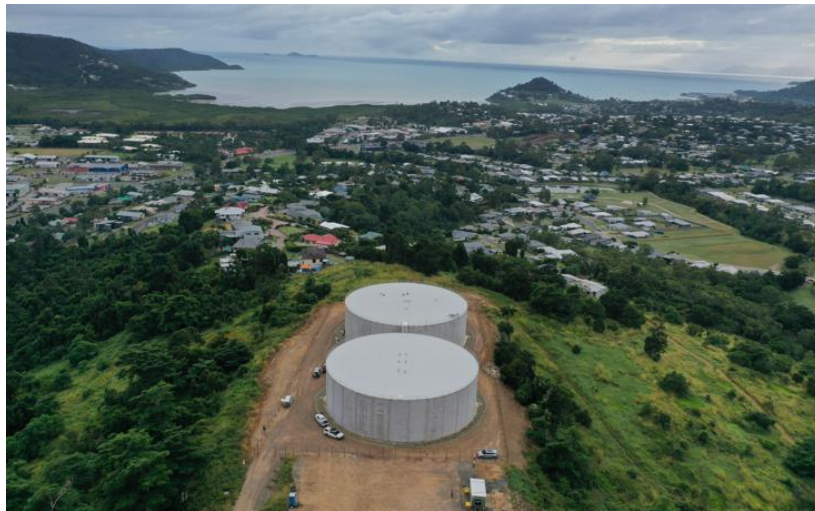
Cannon Valley Reservoir Site – aerial
