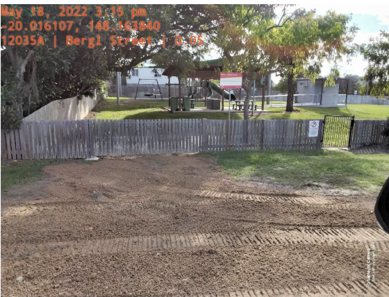
Bergl Street – Scour Repair
