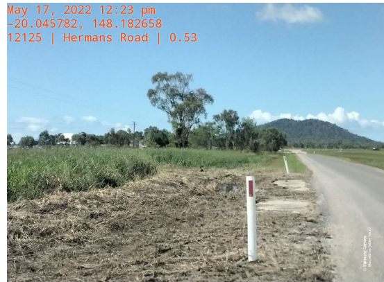
Hermans Road – Culvert Cleaning
