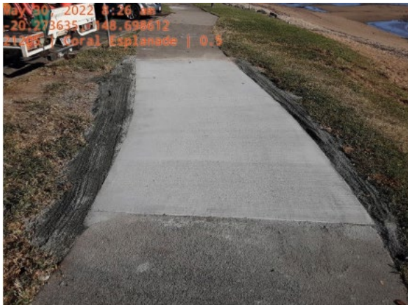
Coral Esplanade footpath replacement
