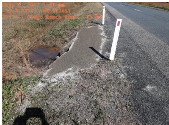
Shoulder repairs on Dingo Beach Road
