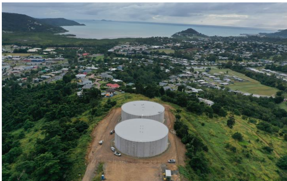
Cannon Valley Reservoir Site – aerial
