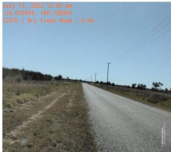
Dry Creek Road – Slashing
