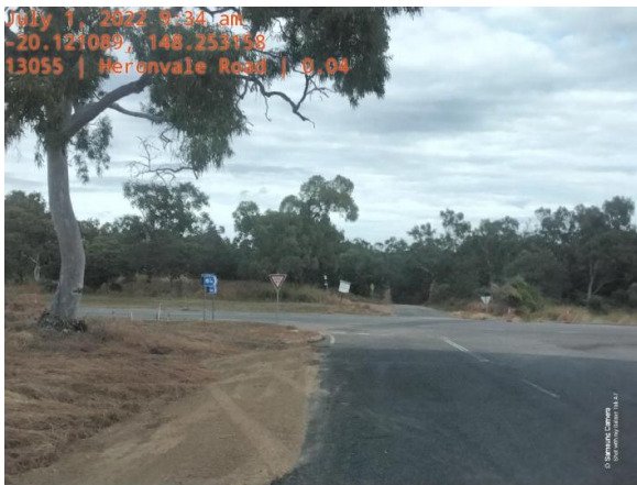
Heronvale Road – Edge Repair
