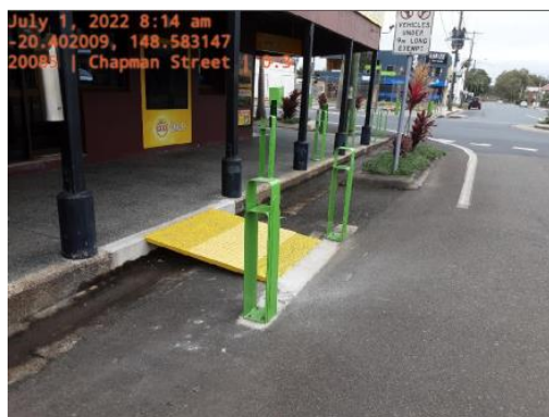
Replaced bollard near the Metropole hotel
