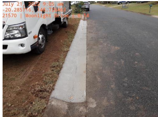
Kerb replacement Moonlight Drive
