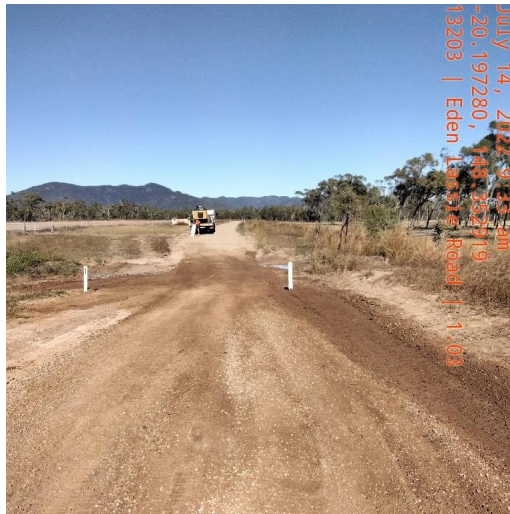
Eden Lassie – Scour Repair
