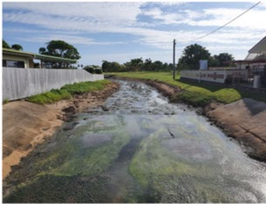
Tollington Road Drain
