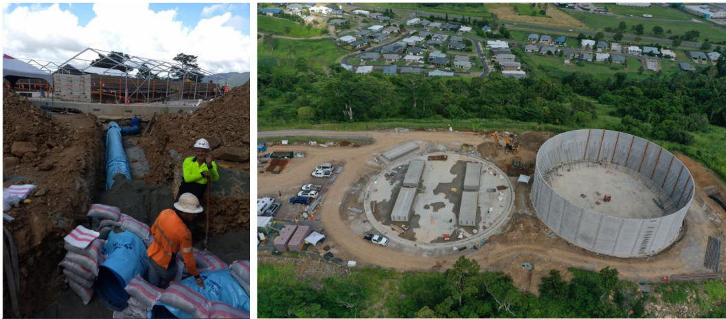
Cannon Valley Reservoir Site – Scour pipe installation + aerial
