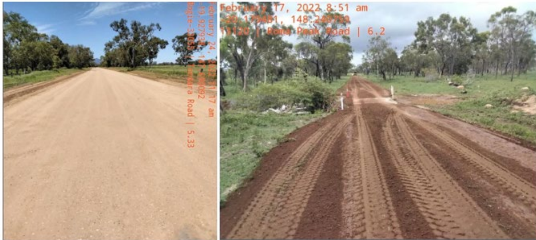
Tondara Road Grading
