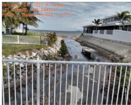
Thomas Street Drain
