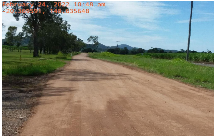
Eckers Road –Grading Works – Maintenance
