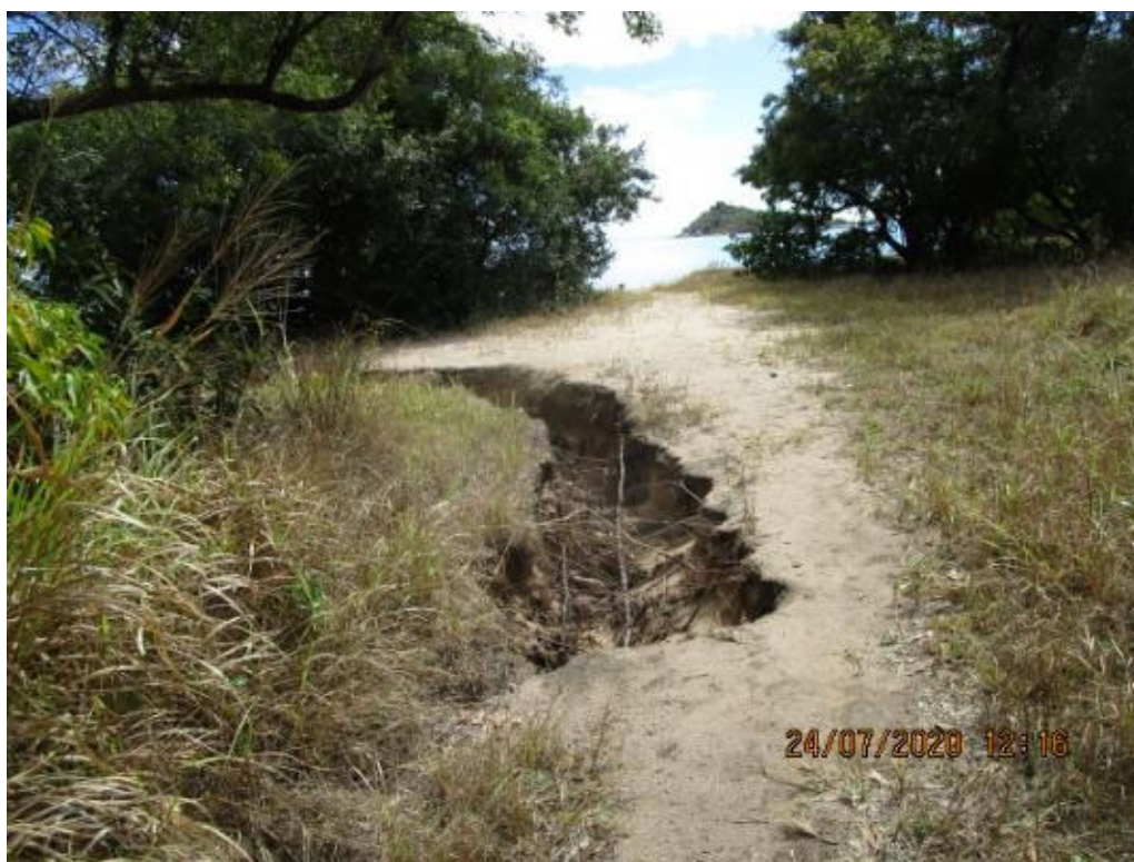
Photo 4: Erosion at Beach 3
