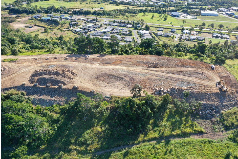
Cannon Valley Reservoir Site – early works package
