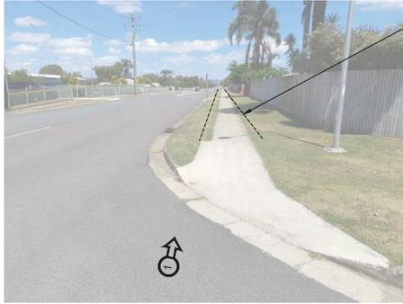
REMOVE EXISTING 1.2m PATH AND REINSTATE WITH NEW 2.5m WIDE PATH
