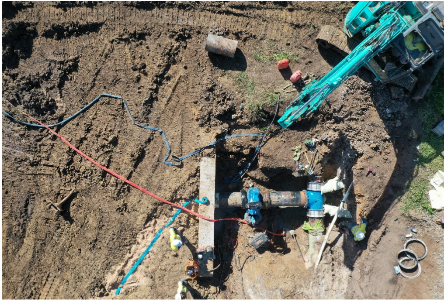
Aitkens Rd - Final water main Cut-In
