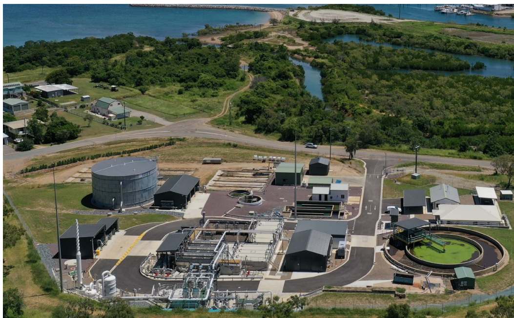
Bowen Sewerage Treatment Plant
