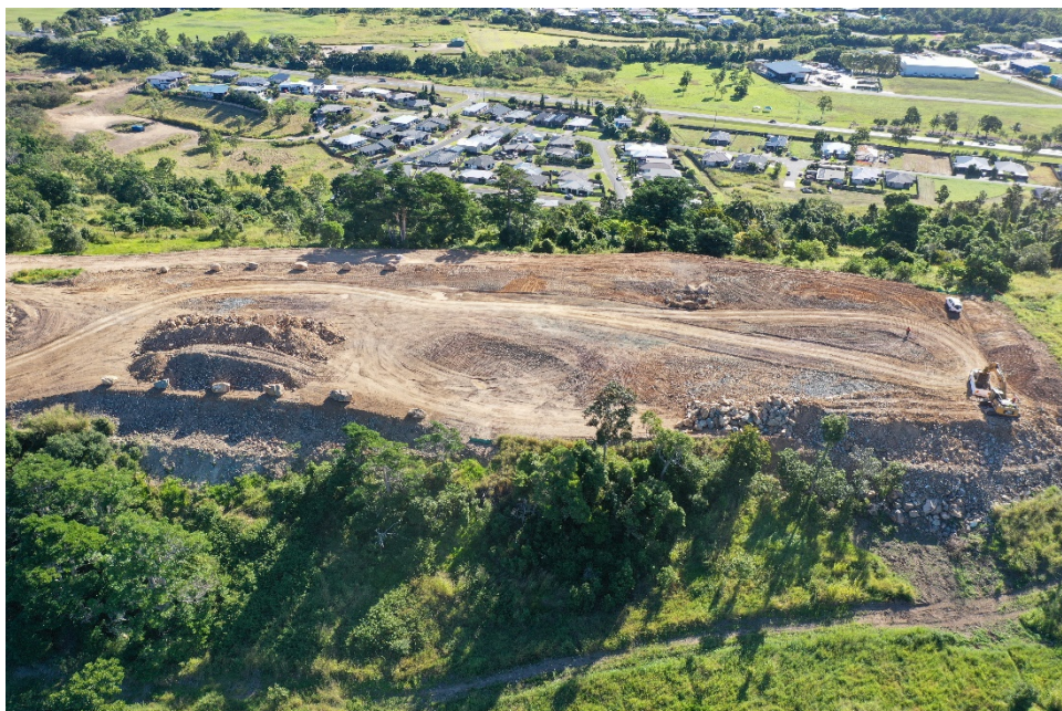
Cannon Valley Reservoir Site – early works package.
