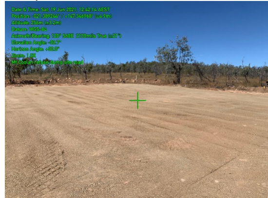
Completed Transfer Site Pad
