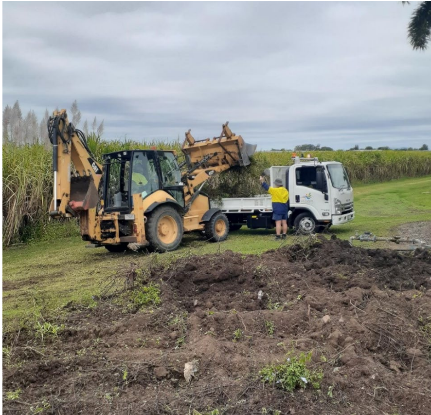
Commencement of the highway garden refurbishment project.
