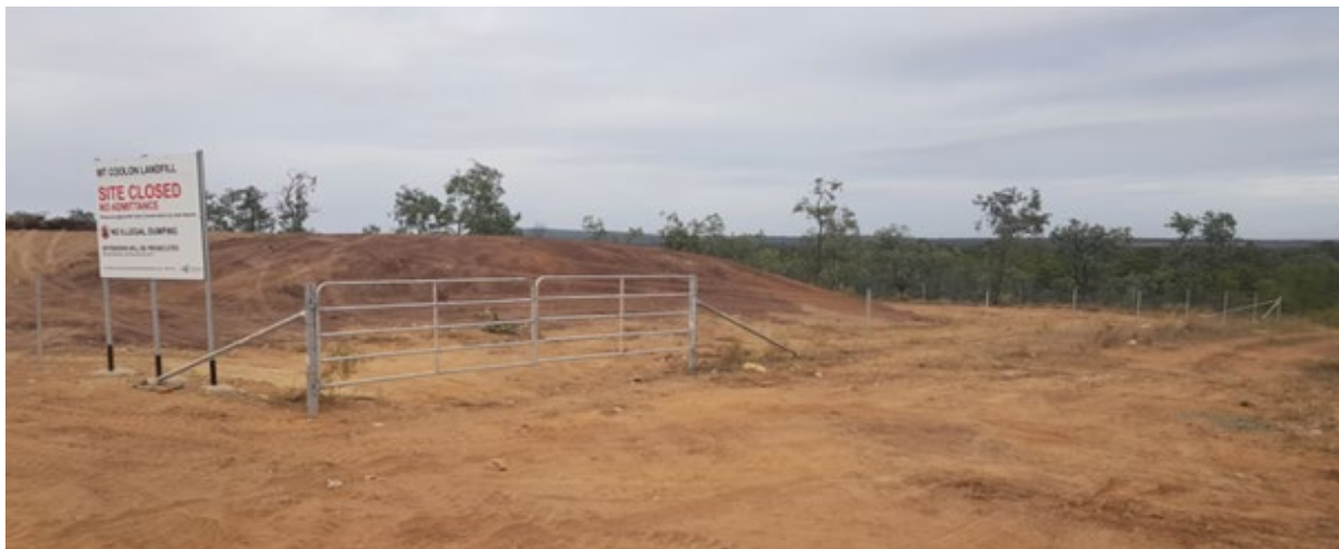
Intermediate capping and closure of Mt Coolon Landfill
