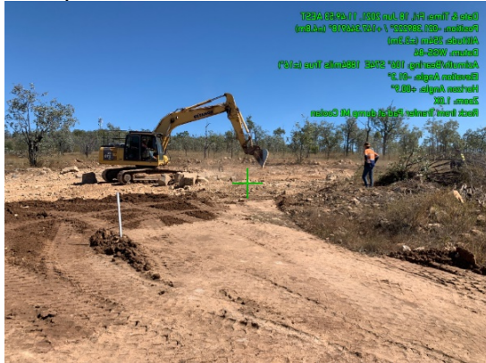
New pad area before
