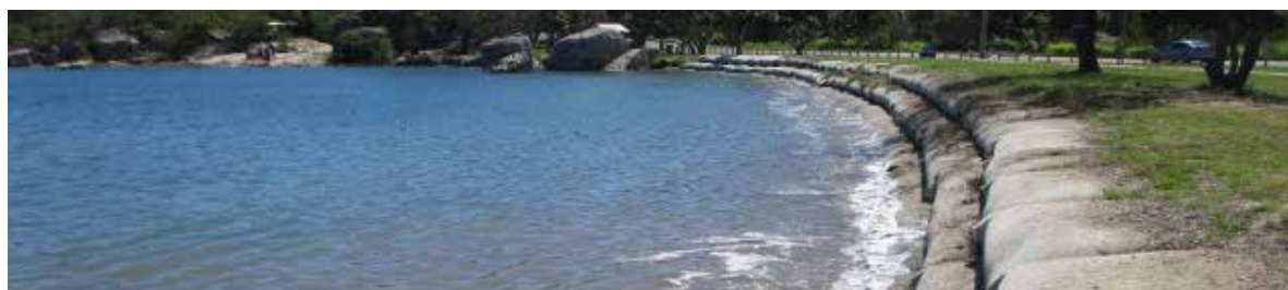
Figure 15: Grays Bay sand bag wall
