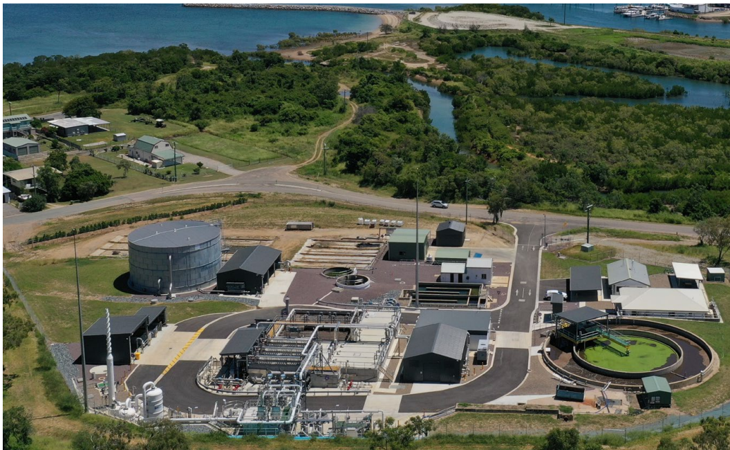
Bowen Sewerage Treatment Plant
