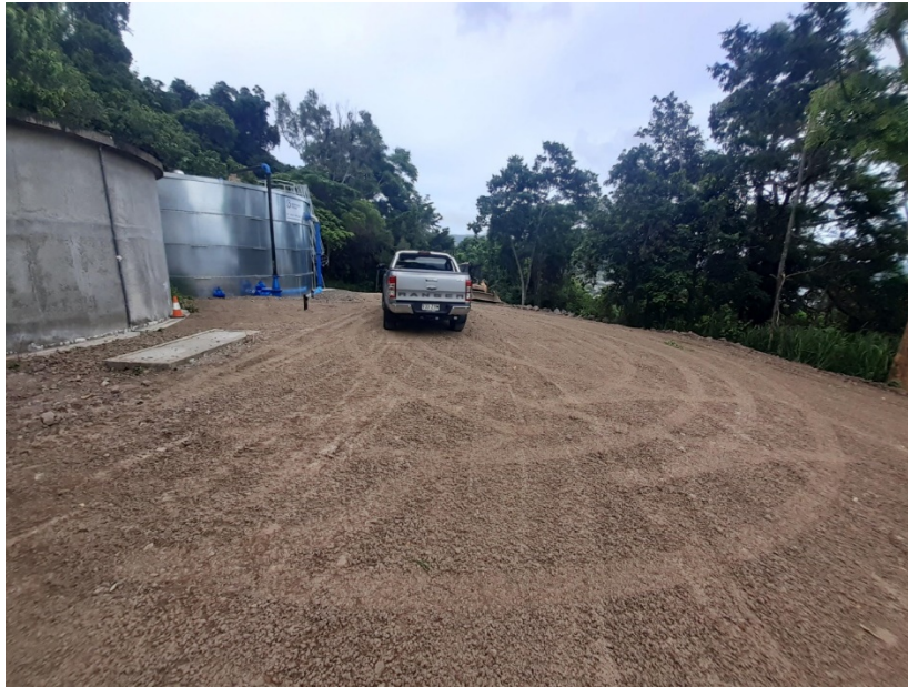
Final site works Coyne Road reservoir.
