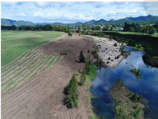
Figure 12: Mary River Project before planting in 2016
