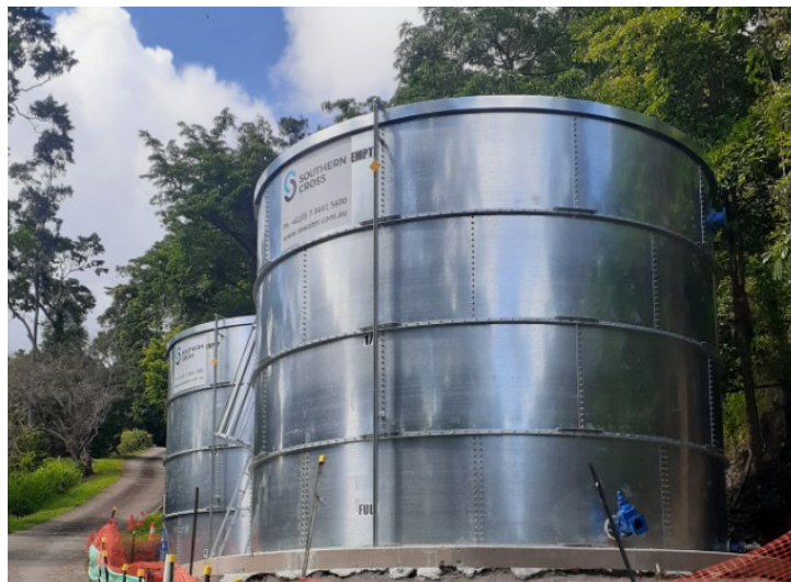
New tanks installed at Moonlight Drive site
