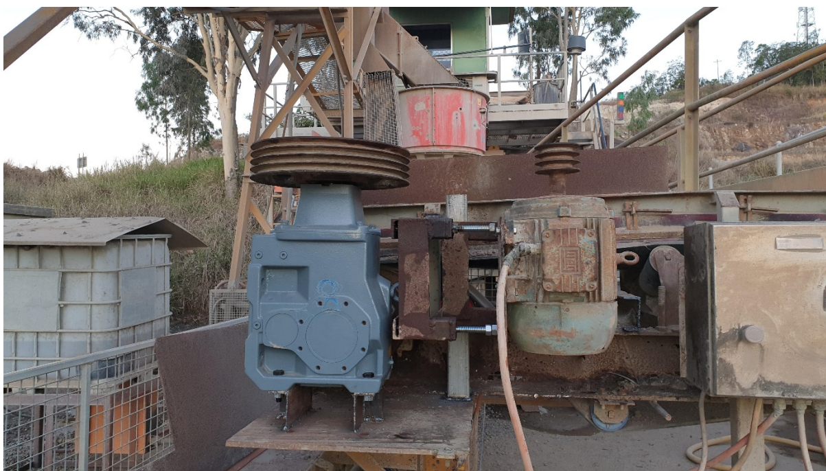
Fig 3. Replacement of the additive bin transmission drive.
