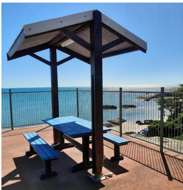
Upgraded the old timber picnic table to a recycled plastic setting. More durable in a seaside location.
