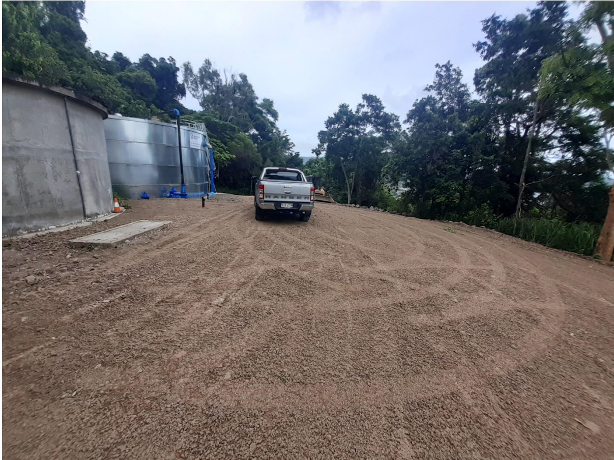
Final site works Coyne Road reservoir.
