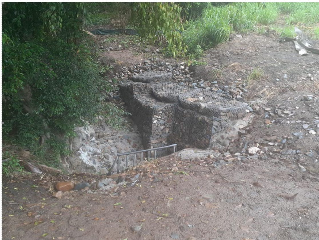
CWNA Stage 1A: Rock Gabion wall installed for scour protection.
