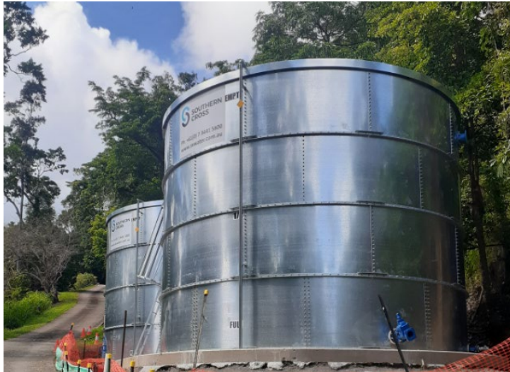
New tanks installed at Moonlight Drive site
