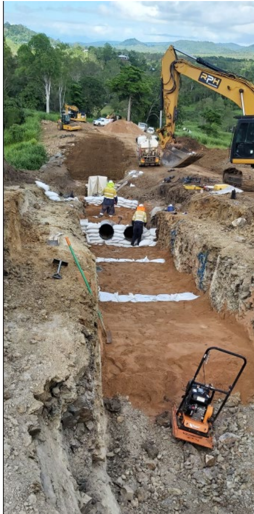
Pipeline Project – Cannon Valley reservoir inlet/outlet pipeline works commenced.
