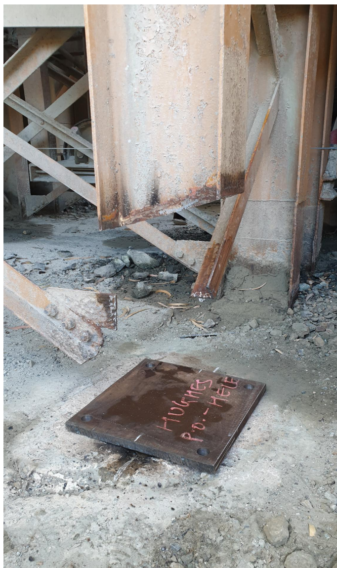
Fig 1 New Foot Plate and Structural Leg Replacement in Progress
