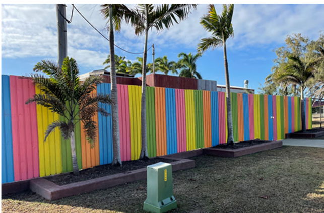
Photo 5: Painted Fence - Bowen Swimming Pool
