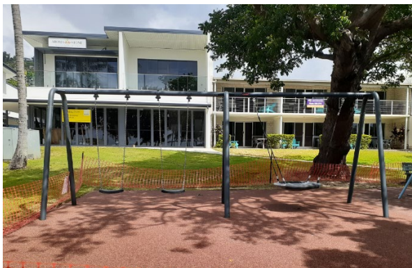
Fairy Tree Park Swing Installation
