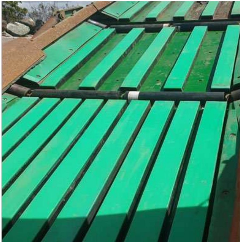
Fig 3 New Impact Bed installed on Foxdale Reclaimer
