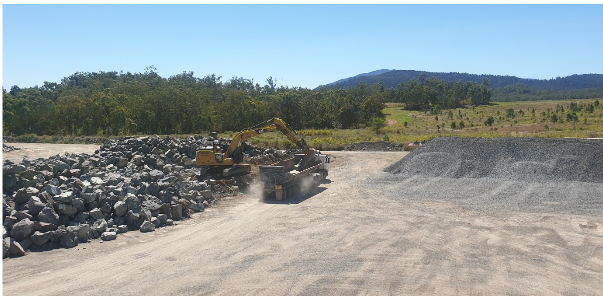
Fig 1 - Excavator loading Large Armour
