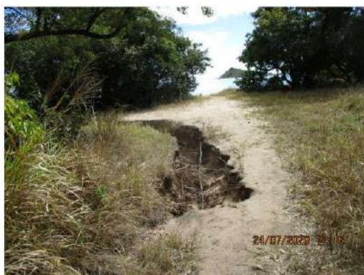
Photo 4. Erosion at beach 3.
