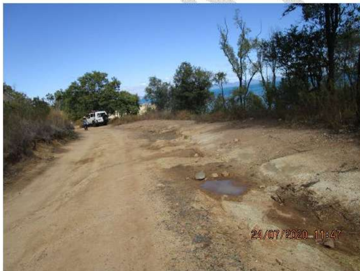
Figure 8. Showing erosion caused by vehicle access to the beach.
