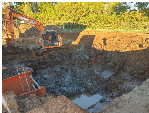
Excavation works for the emergency storage tanks
