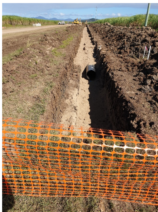
Main works in progress
