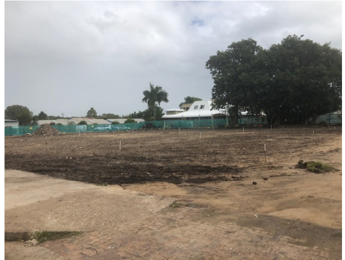
PEC site post demolition
