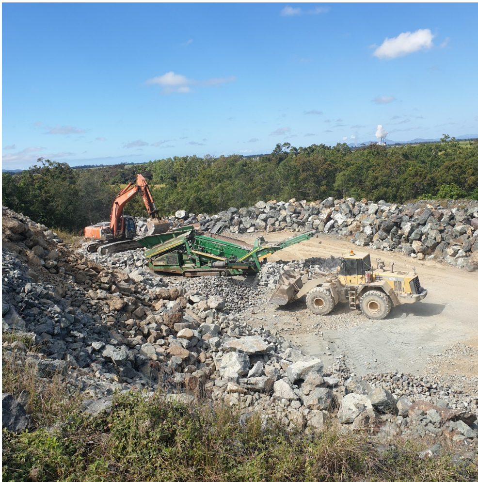
Photo – Production of small armour rock
