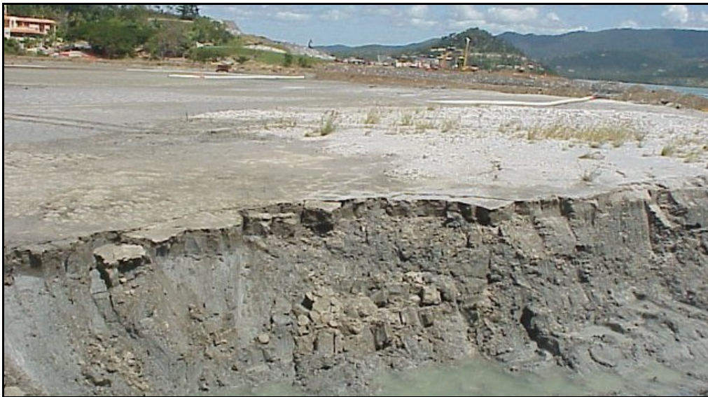
Photograph 12. Dredged PASS used for land reclamation at the Abel Point marina, S DL map unit
