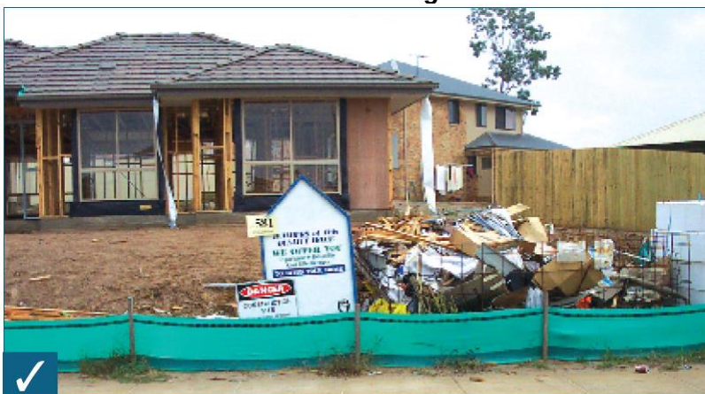
Sediment fence and best practice building site
