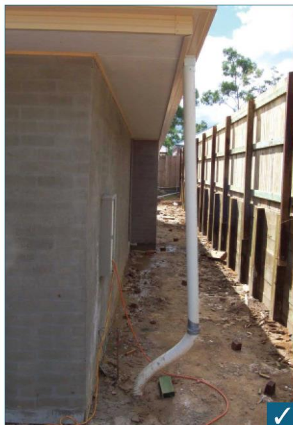
Temporary roof water connection
