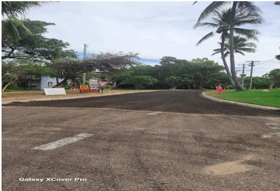
Project: 4262 Mackenzie Street Kerb & Channel
