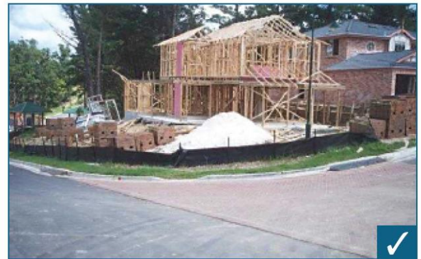
Effective on-site erosion and sediment control
