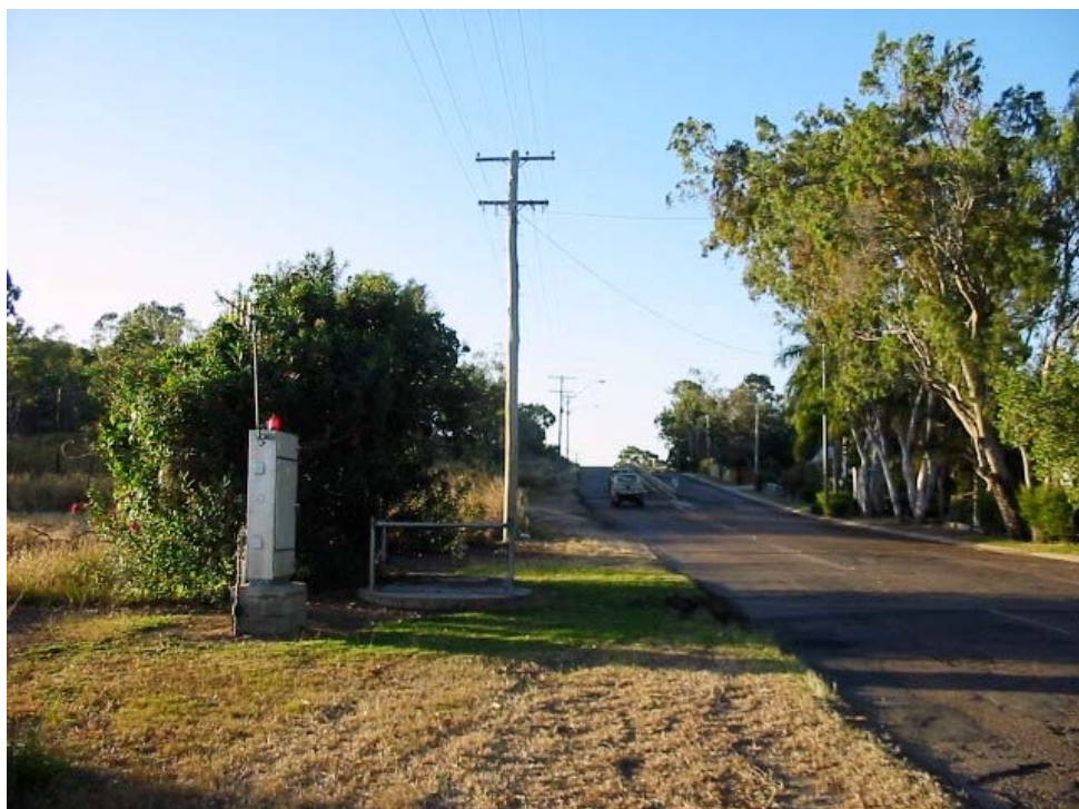
Plate 8: Sewage Pump Station in low lying area on Mt Nutt Road
