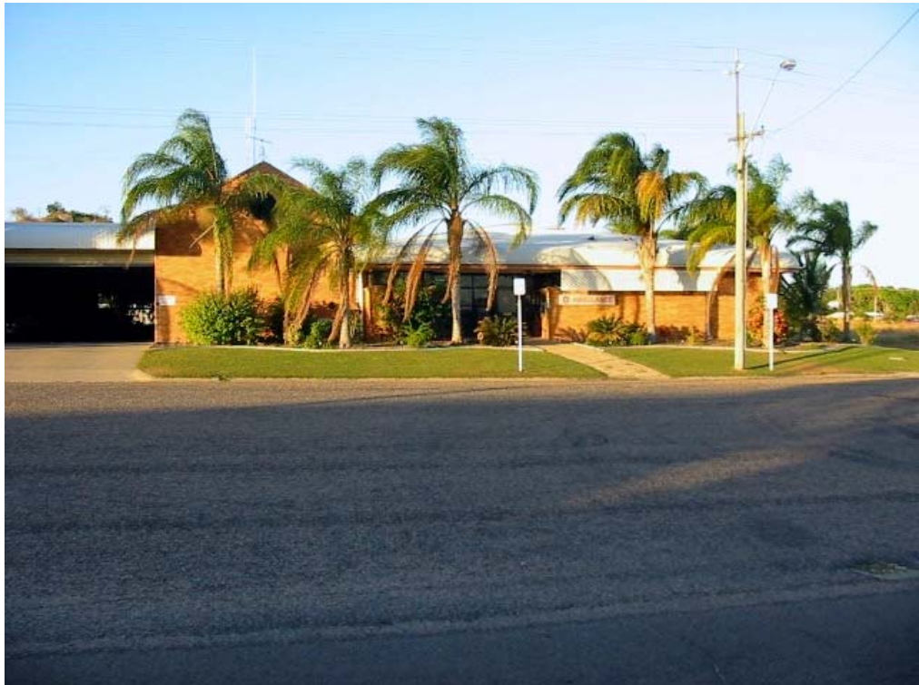
Plate 10: Ambulance Station, John Street
