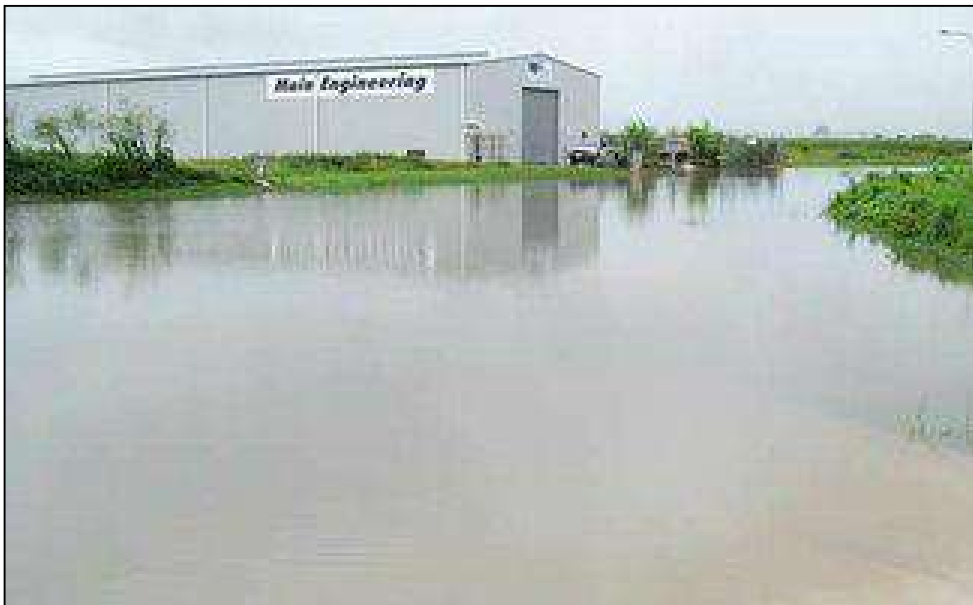
Figure 16 March 2011 Event – Flooding at Horsford Place
